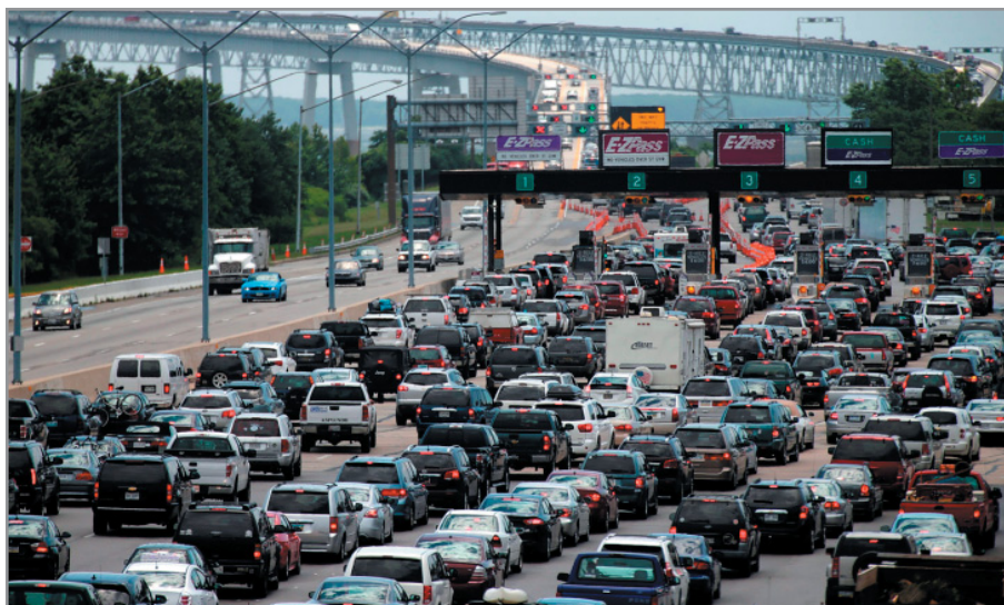
Chesapeake Bay Bridge, 2013. 14
